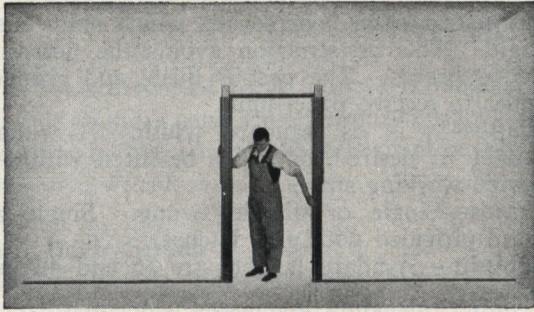
Setting Door Posts
